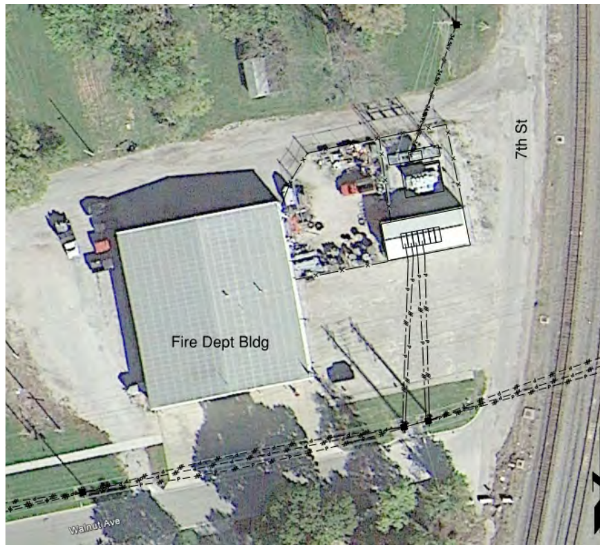
Figure 1: Existing 7 th St Substation Site.
