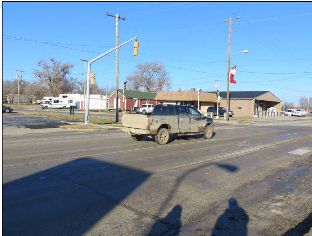
Figure 8 - Pavement Markings from South of the Southeast Corner of the Intersection Looking Northwest (6th St. & W. Pacific Ave.)
