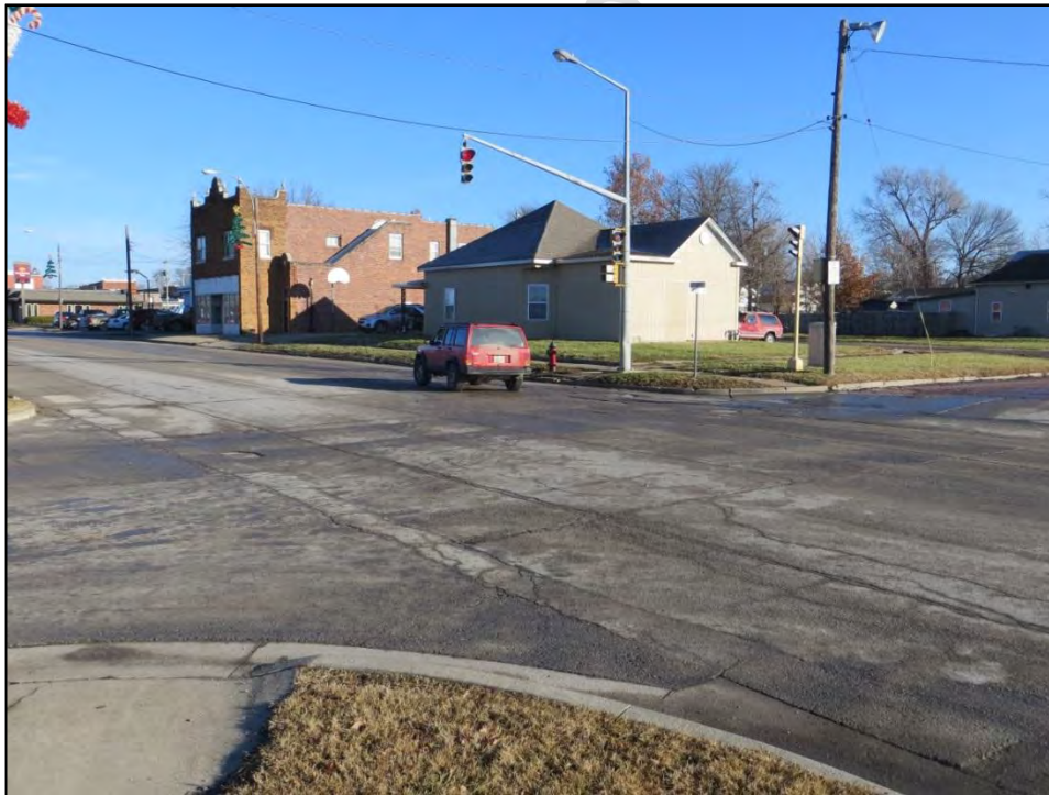
Figure 14 - Southwest Corner Looking Northeast (6th St. & W. Pacific Ave.)
