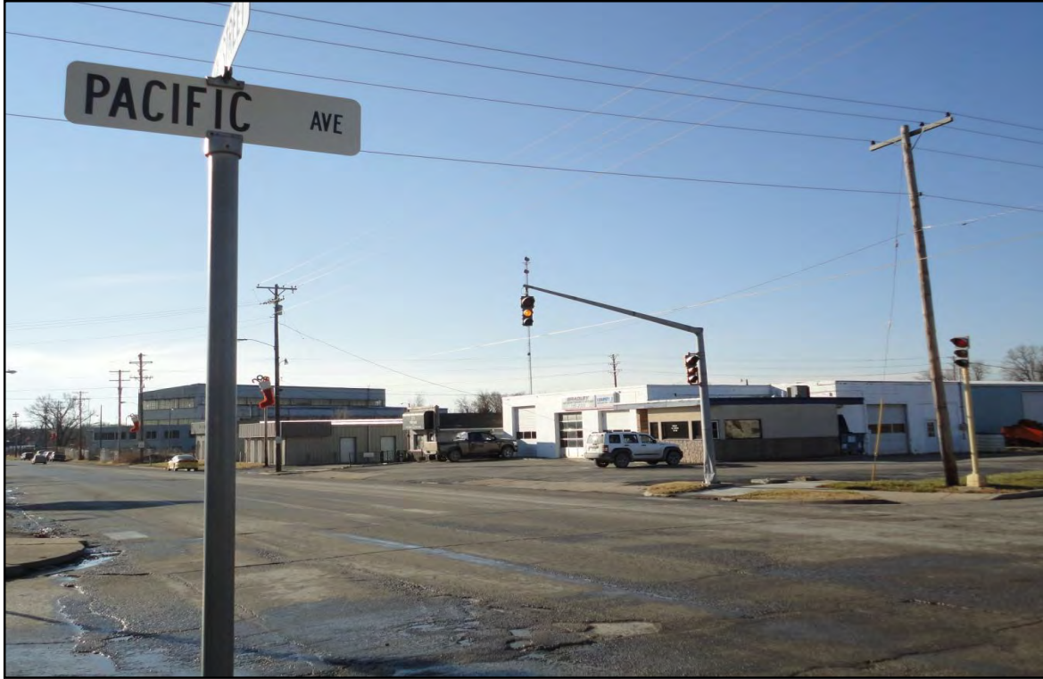
Figure 3 - Southbound Signal Mounted on Mast Arm (6th St. & W. Pacific Ave).
