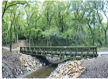
Bridge Replacement at Ernie Miller Nature Center
