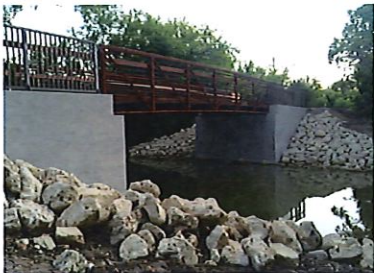
Andover Road Pedestrian Bridge
