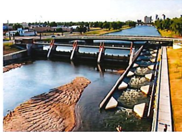
Lincoln Street Bridge and Dam
