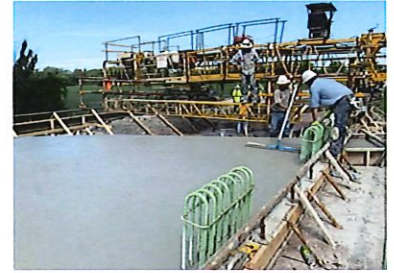
Bridge FAS 390 Replacement
