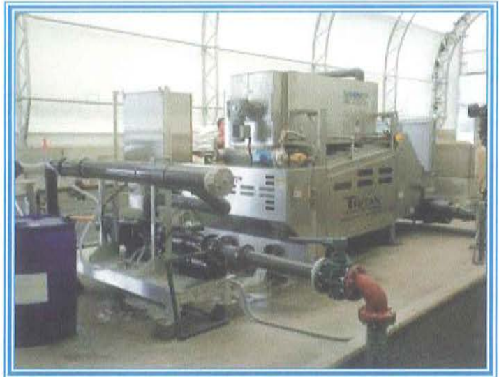
The TRITAN discharges a biosolids cake with a solids concentration of 15 percent to 20 percent.
