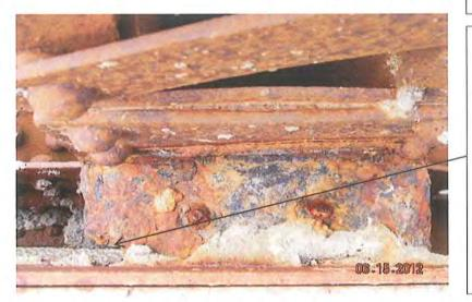
"Zipper" rust in outside purlins. Essentially the bottom flange of the I-Beam is un-zipping from the web. This is consistent along both outside edges of the bridge and is likely due to deicing salt spilling over the edge of the deck over time.
