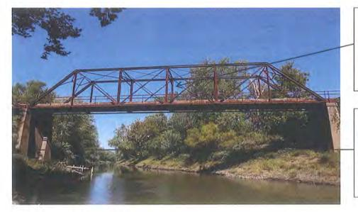
Superstructure for this bridge includes the Steel Truss Members, Concrete Bridge Deck, and Bridge Bearing Assemblies.
