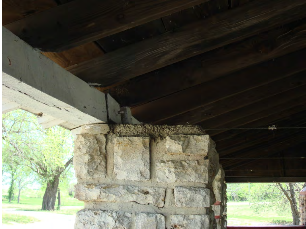
Timber beams installed on the outer edge of the piers
