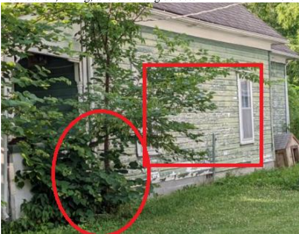
Protective treatment defects, woody vegetation around structure
