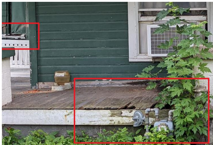
Porch decking, windowsill defects
