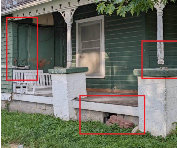
Foundation, siding, and overhang defects
