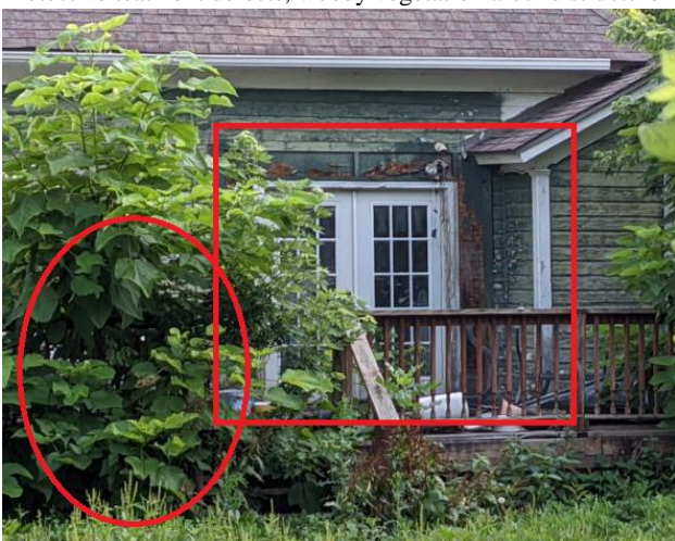
Siding defects, vegetation encroachment on structure.
