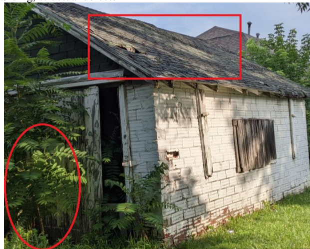
Detached structure nuisance, roof and siding defects and coatings
