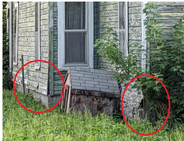
Siding, structural defects
